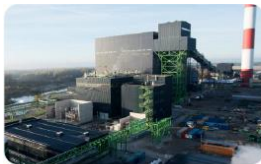
Auvere Power Plant
